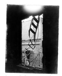
The Triangle Shirtwaist Factory's only fire escape collapsed in a blaze that killed 146 workers and spurred labor reforms. *Kheel Center, Cornell University*
